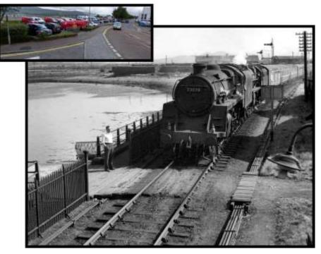
This 1955 image was taken from the signal box and shows the fishermen's crossing and boat slip. When the railway was being planned, fishermen and boat owners had objected strongly to the route along the foreshore. This crossing helped mitigate their loss of direct access to the sea.
