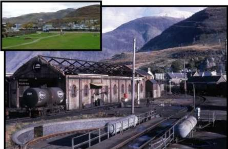
This 1964 view shows the turntable and engine shed, looking the worse for wear towards the end of its life.
