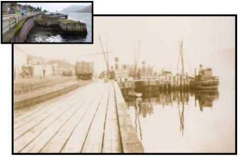
This image shows the 'New Pier' and the two quayside sidings which served it. After the distillery traffic diminished, one siding was removed but the line nearest the sea was retained to stable coaches and to allow locos of arriving services to draw forward (to avoid blocking access to the Town Pier for too long).
